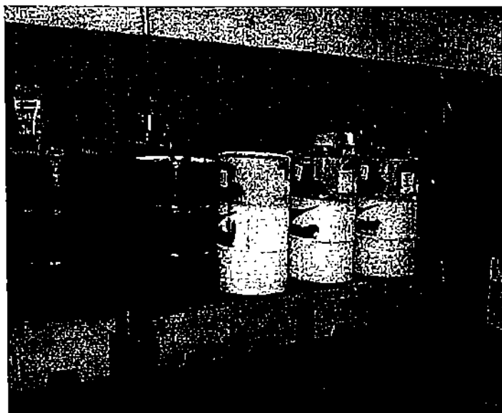
Figure 2 - Drums stored indoors on spill pallet.
